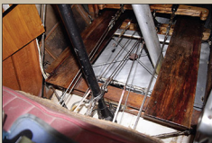
The bracing wires and control cables make for a rather cluttered appearance between the foot boards (F14) and empty shell chute from its single gun. Note the aluminium and linen areas of the fuselage bottom.
