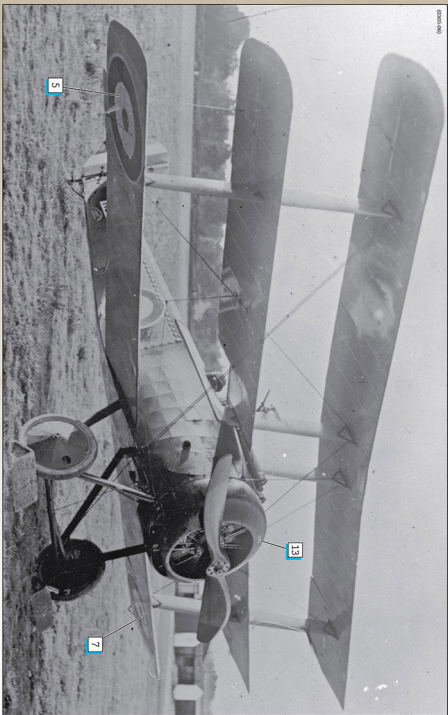
An unidentified twin gun Sopwith Triplane from the same September 1916 Clayton & Shurtleworth production order as N533. Despite only 6 aircraft being produced, this aircraft differs from N533 in that it is fitted with a Kotherham petrol pump, retains its factory stenciling under the starboard serial number and has an oval hatch in the side cowling. Note the cockpits with a white outline under the wings which are believed to be peculiar to these late production Clayton & Shurtleworth built twin Vickers armed Tripes and the white aileron control horns.
