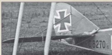
Tailplane detail from crashed Rumpler C.IV 8270/16 as seen on page 13. Note the factory work number (wn), possibly 1691 or 1681, stenciled onto the fin and rudder and R.U. (Rechts Unterstutzen) [56] above the "right under strut" attachment. The sharp "saw tooth" edges on the bottom strut [D10] were intended to prevent ground crew from using these struts to lift the aircraft. The broken tail skid rests on top of the tailplane.
