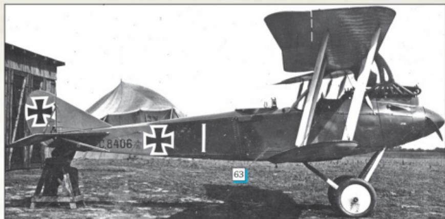
Rumpler C.IV 8406/16 T from the 3rd production batch of 150 aircraft ordered in November 1916 displays many typical early production features; full length fuselage fabric, small form of weight table, fully faired elevator control cables and sleek propeller spinner.
