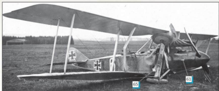
Rumpler C.IV 8270/16 has landed heavily destroying the undercarriage, propeller and starboard lower wing. It would appear **13** that 8270/16 was from the 1st production batch of 100 Rumpler C.IVs ordered in September 1916.
