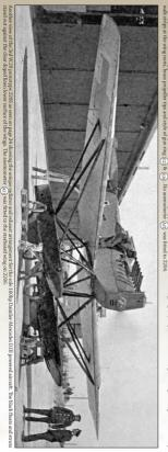
totype W.29 2204 resting peacefully at the beach. The ribtapes on the underside of the wings appear to have had an additi-k strips at the wing roots, brass propeller tips and style of gun ring  $(v_{12})$  &  $(v_{12})$  . No anemometer  $(\lambda_2)$  was fitted to 2204. ossy dope which is reflecting the background light. Note non-slip
