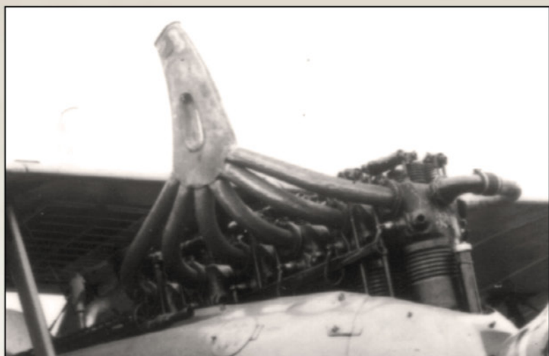
Close up of w/n 4821 showing exhaust details (via Colin Owers).
