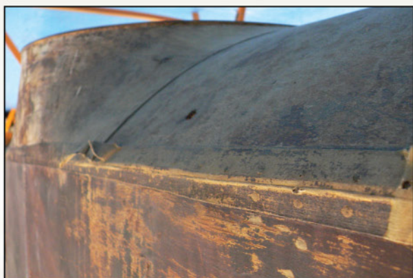
Detail of the reinforcing tape applied to the edges of the fuselage. These often appear quite dark in contemporary photos compared to the surrounding fuselage colour (Memorial Flight Association).
