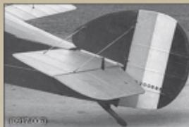
Fin and rudder detail from the unidentified Ruston & Proctor built Sopwith E.1 Camel seen on page 12. There were several variations of elevator control cable exit points in the fuselage depending on the manufacturer.
